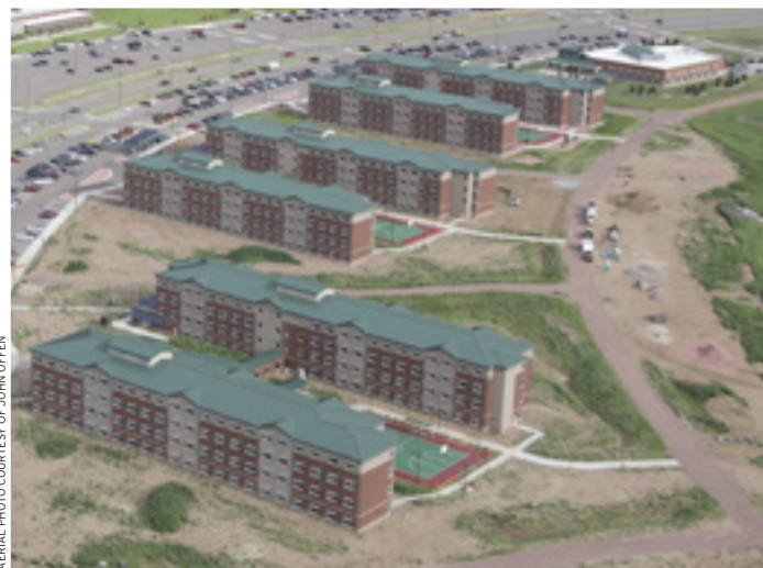
AERIAL PHOTO COURTESY OF JOHN OFFEN
