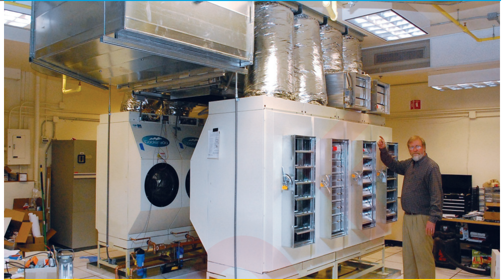
The above photo shows the Coolerado units installed at the National Snow and Ice Data center in May 2011. Photo used with permission from the National Snow and Ice Data Center.
